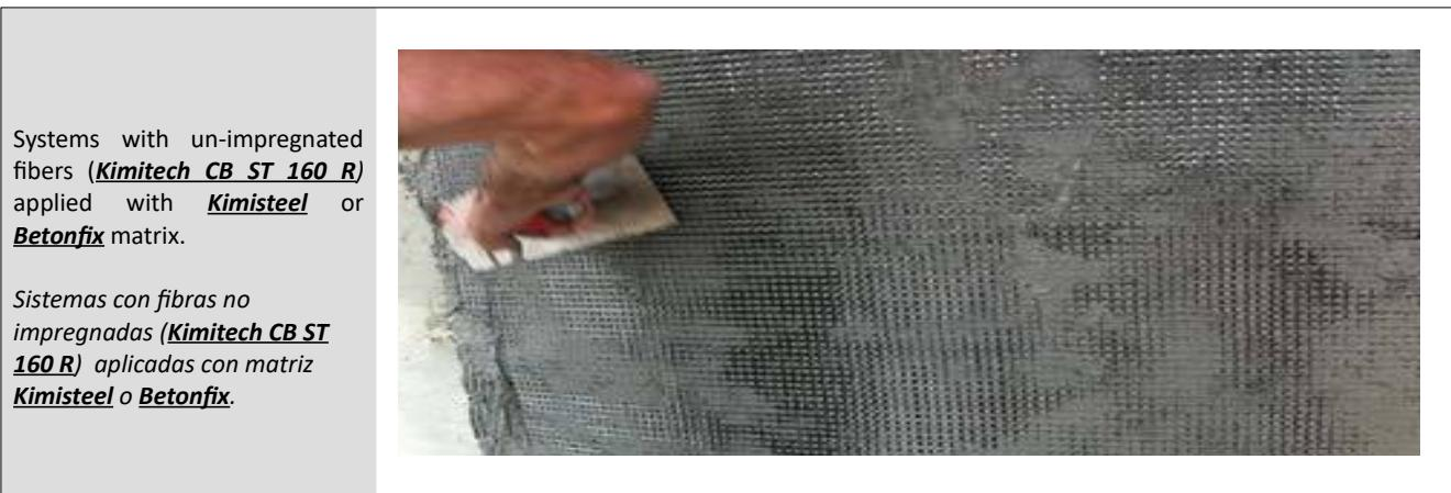
Systems with grids of impregnated fibers applied with lime-based or cementitious mortars, connected to the substrate through connectors.
